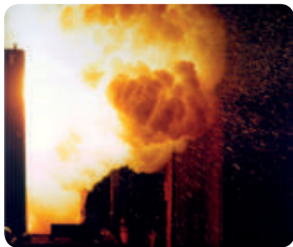
Switchgear explosion due to arc fault
